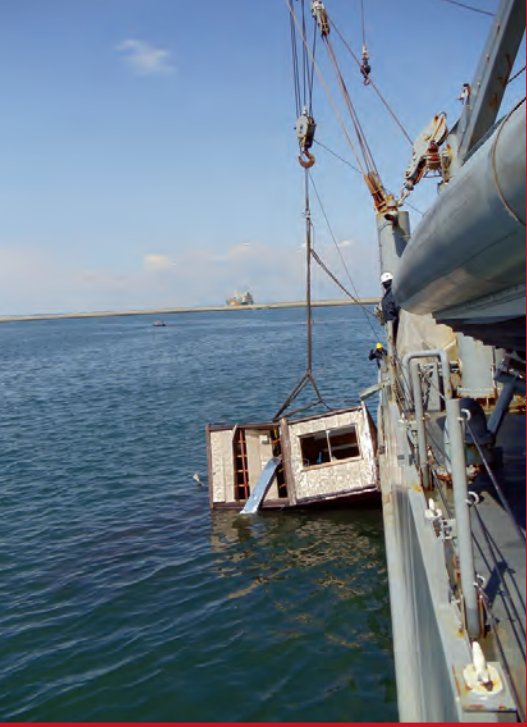
Debris removal on USNS SAFEGUARD in Hachinohe. (By: MDV Jon Klukas)
